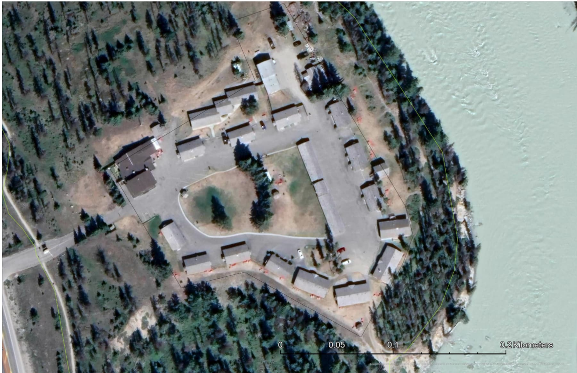
Figure 60: View of the Jasper House Bungalows property pre-fire. Only the maintenance structure on the top middle and main structure in the top left have asphalt shingles. The rest of the structures have wood shake roofs.
