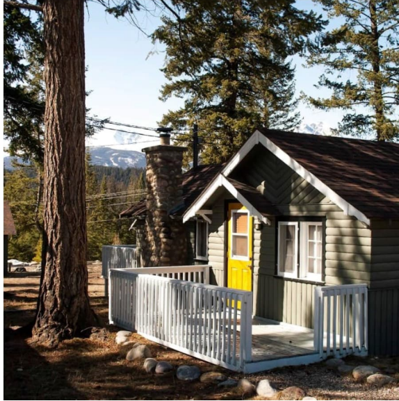
Figure 40: Image from Tekarra Lodge Facebook page showing pre-fire fuel conditions around the southwest side of the property.
