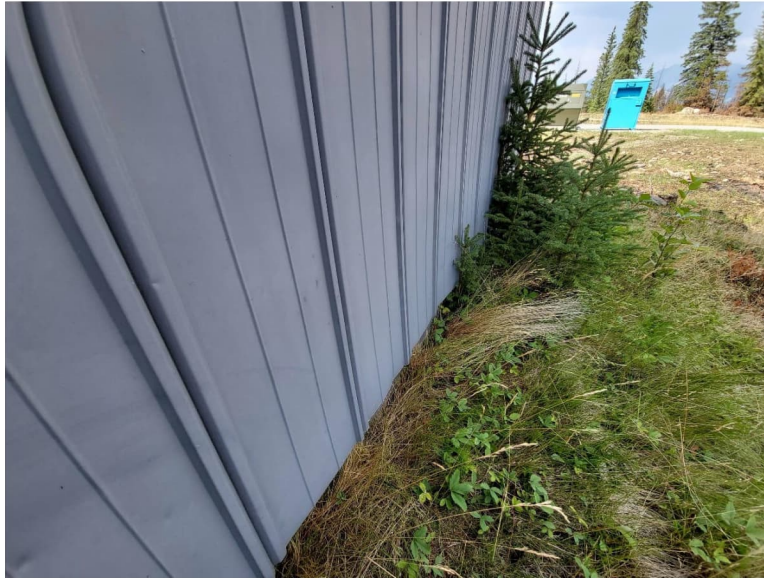
Figure 50: Unburned cook shelter in Whistlers campground with similar spruce fuels growing near its base.
