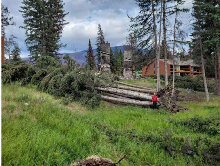
Figure 25: View looking east of the burned structure just northeast of Beauvert Lake at Jasper Park Lodge.
