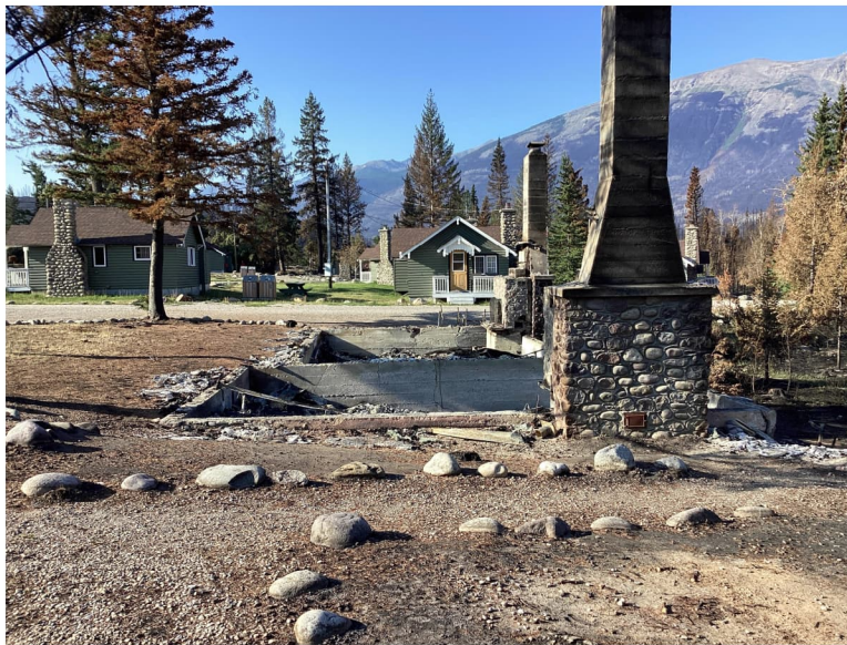
Figure 41: Looking south from the northwest side of Tekarra Lodge. The burned structures were built similarly to the two seen in the background.
