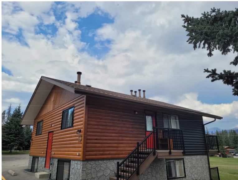
Figure 46: Structure with visible damage (yellow structure on the area map) adjacent to the burned structures.
