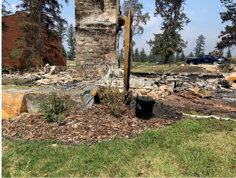
Figure 27: Vulnerability (mulch bed with fence attached to structure) present on the burned structure on the shore of Beauvert Lake.
