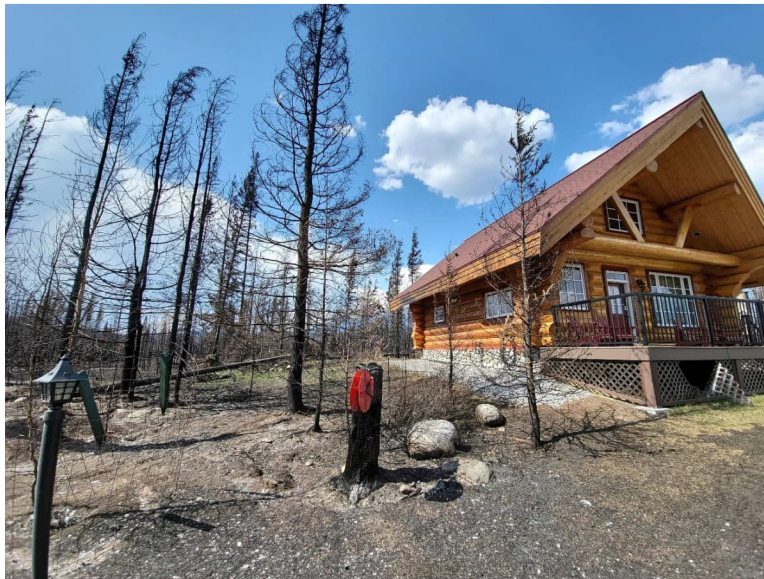
Figure 38: Close view of the side of the unburned structure showing the direction fire approached from.
