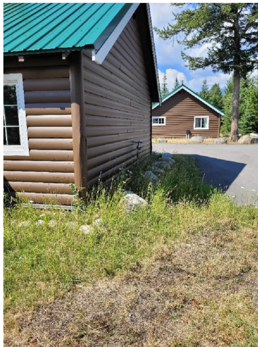
Figure 59: Typical fuel around the Pine Bungalows.
