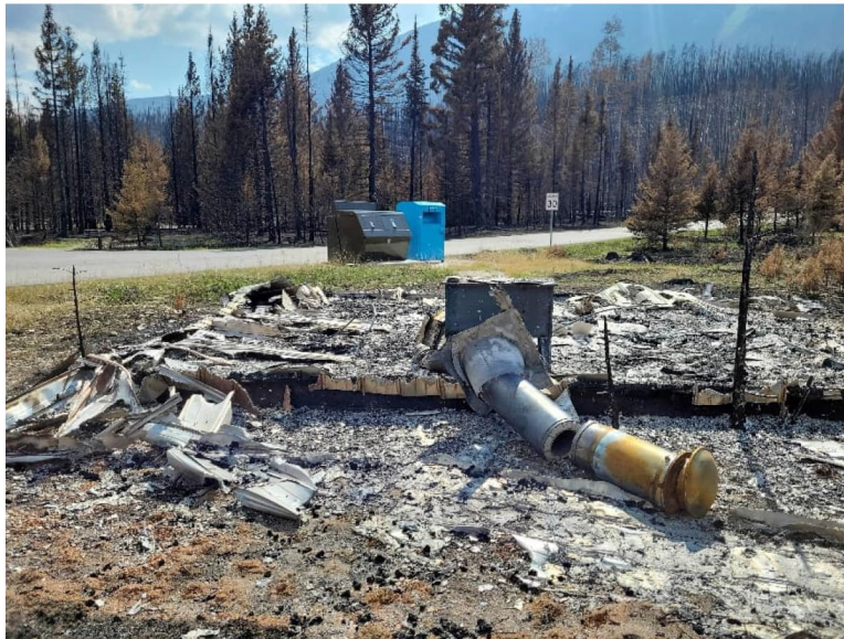
Figure 49: Burned cook shelter in Whistlers campground showing spruce seedlings and saplings growing up against structure.
