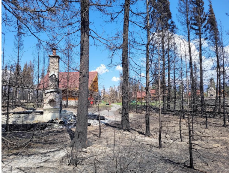
Figure 37: Burned pair to the unburned structure on the southwest side of the property.
