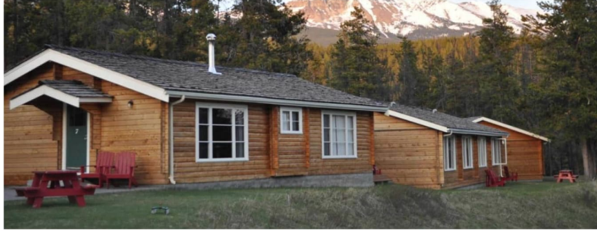
Figure 61: Picture from Jasper House Bungalows Facebook page showing the pre-fire condition and structure characteristics of the cabins.
