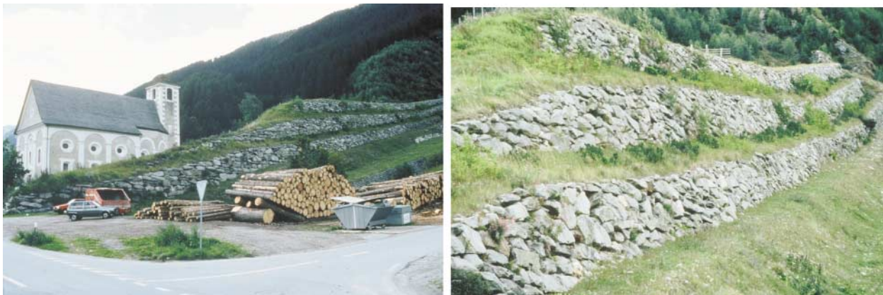
Fig. 9. Snow avalanche berm in Switzerland (courtesy, Dr. Steiner, Bern, Switzerland).
