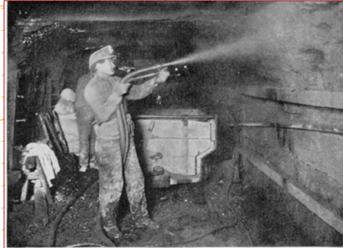
Photograph from U. S. Bureau of Mines LINING A MINE WALL WITH ARTIFICIAL ROCK
