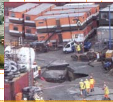
The 1994 Heathrow tunnel collapse, a NATM tunnel in London Clays.
