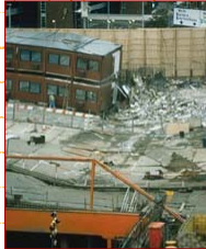
The 1994 Heathrow tunnel collapse, a NATM tunnel in London Clays.
