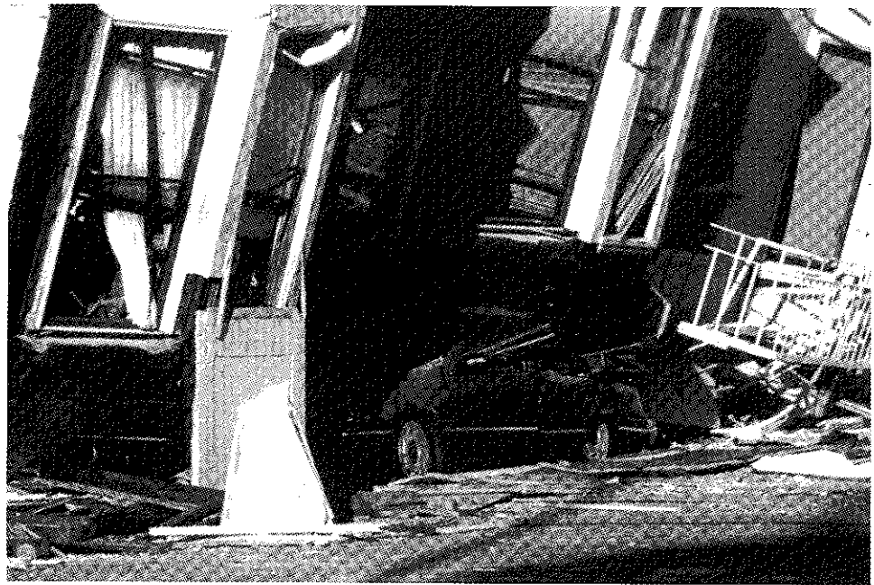
Figure 1.17 Damage to buildings in the Marina District of San Francisco resulting from the 1989 earthquake. (Photograph courtesy of John K. Nakata, U.S. Geological Survey.)
