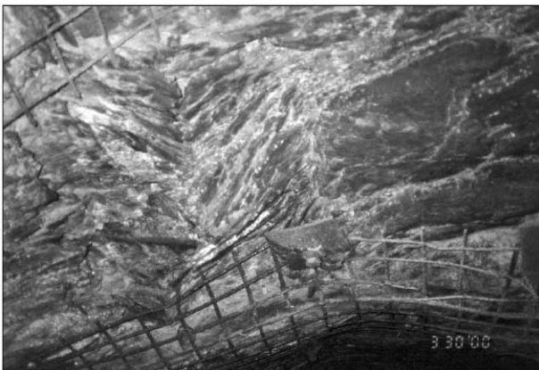
Fig. 15. Stress-induced breakout and notch formation along the roof of the Furka access tunnel "Fenster Bedretto".
