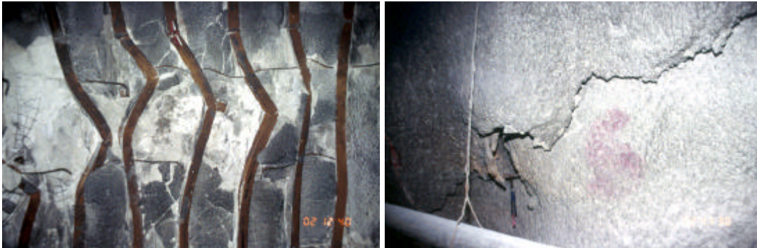
Figure 4. Buckling and bending of 150x150 mm steel ribs with steel lining between crown and right spring line (LEFT). Shearing of shotcrete lining along left bench (RIGHT).
