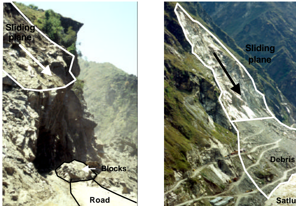
Figure 3. Blocking of the Hindustan-Tibet-Highway by a rock fall (LEFT). Rock slide at the dam site blocking the Satluj River (RIGHT).
