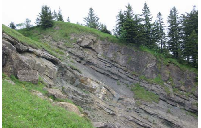
Figure 1. Lateral release margin at the top of the Goldau rockslide showing interbedded conglomerates and marls dipping at angles between 15° and 30°.
