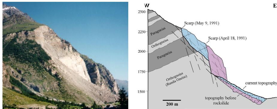
Figure 5. The 1991 Randa Rockslide illustrating the two key sliding events (after Schindler et al. 1993)
