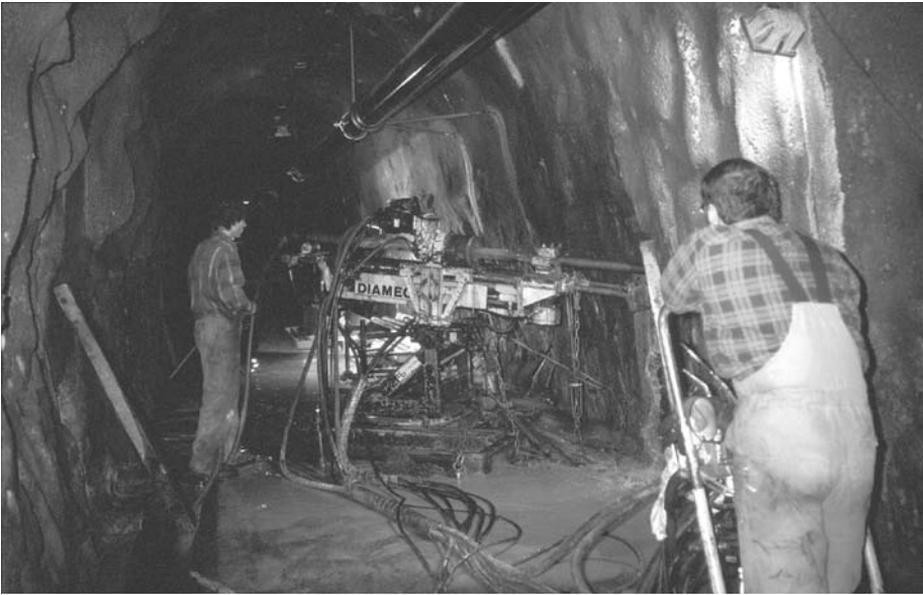
**Fig. 7.** Sub-horizontal triple-tube drilling normal to the strike and dip of the shear zone
