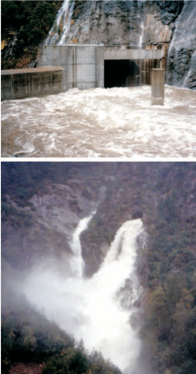
Fig. 3. Photos of diversion tunnel constructed to divert the Rovana River away from the toe of the Campo Vallemaggia landslide (see Fig. 4 for location).
