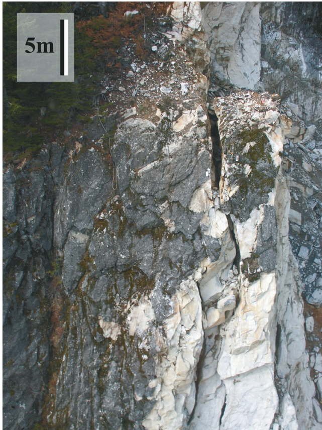
Fig. 11. Photograph showing present-day subvertical open tension cracks behind the back scarp of the 2003 Afternoon Creek rock-slide.
