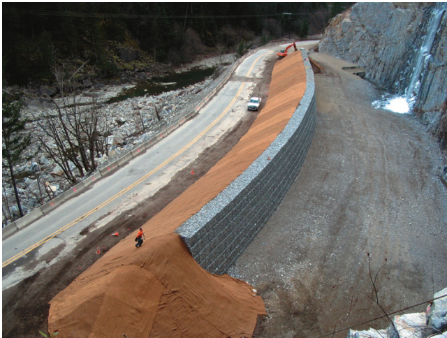
Fig. 21. Protective embayment on Washington State Route 20 at Falls Creek completed in 2006. Photograph courtesy of Tom Badger (Washington State Department of Transportation).
