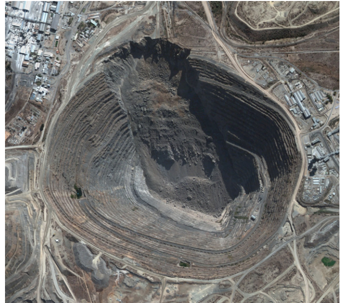
Fig. 2. Quickbird image of the northwest wall failure at Palabora.
