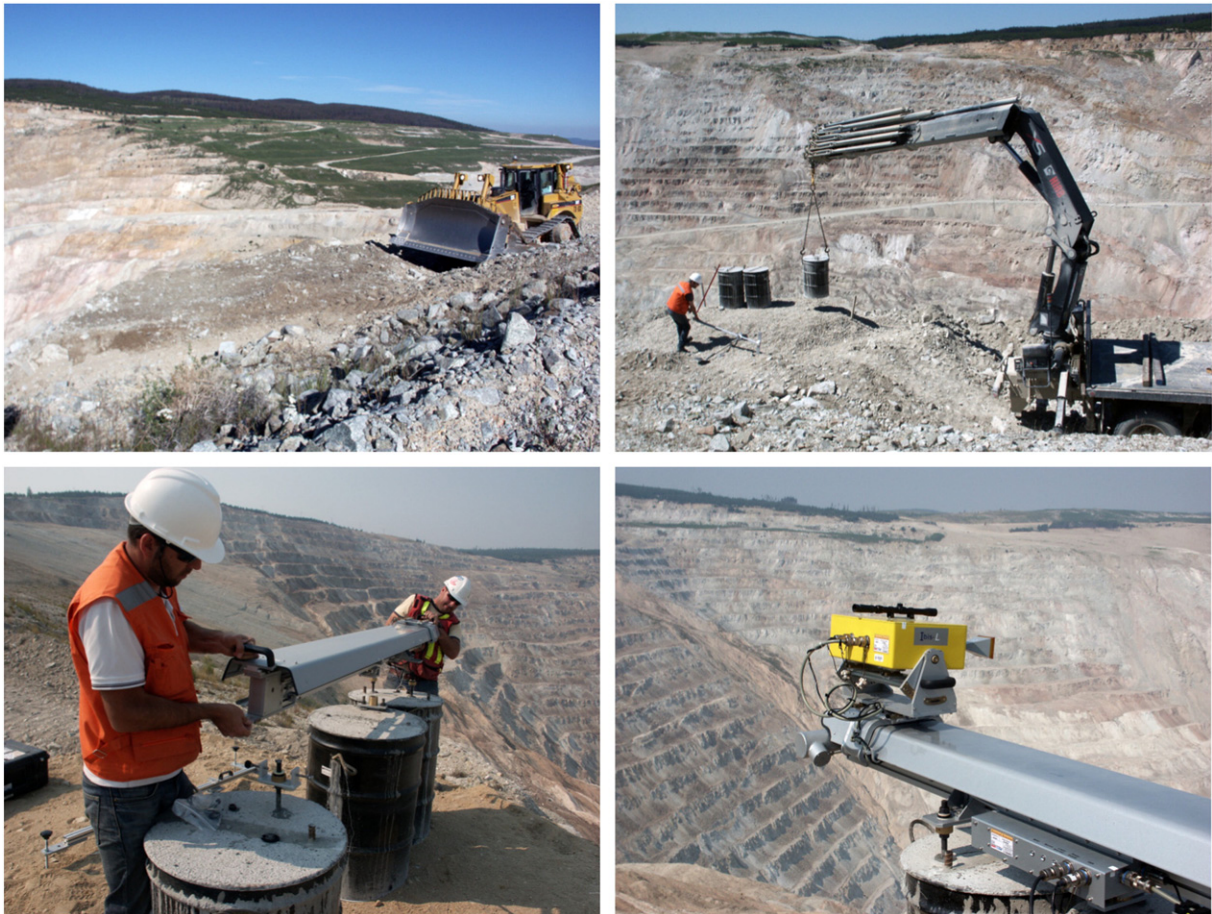
Fig. 4. Site preparation and installation of the IBIS-M radar unit for the 3-D radar experiment, showing: leveling and grading of gravel site pad, lifting of concrete filled drums for radar base, fitting of leveled radar guide rail, and radar positioning for pit wall monitoring.
