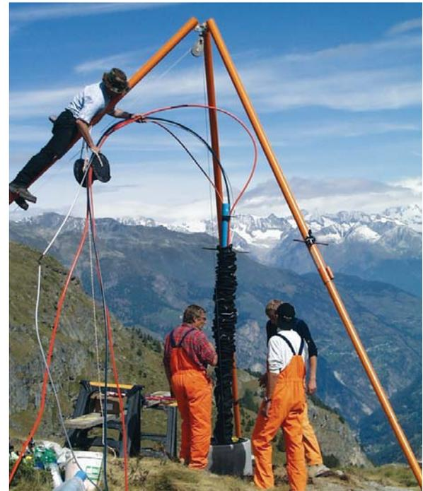
**Installation of borehole instrumentation at the Randa In Situ Rockslide Laboratory**
